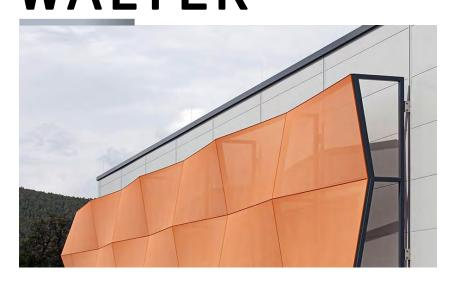
The height was predetermined by a noise protection requirement, as this structure takes on the function of a previously existing noise protection wall.
