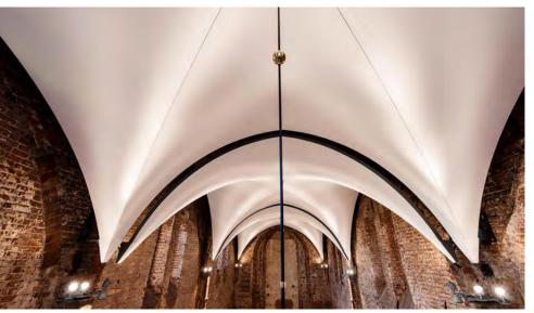
For the new acoustic ceiling, the textile sails were stretched onto an aluminum construction. Each of the self-supporting sail elements is ten by ten meters. The construction of the ceiling, which is only fixed at points on the walls, is unique in Germany.
