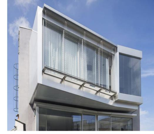
Movable curtains of translucent PVC mesh cover the facade of this block of offices and flats in Paris, which has been converted from a 1970s concrete structure by local practice Moussafir Architectes.
