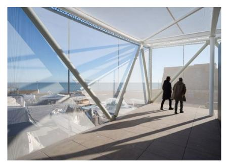
The architectonic structure is covered with wide walls in PVC mesh that allows the light to pass through, creating light and shadow effects during the day.
